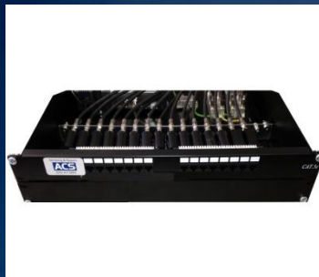
Standard Patch Panel presented at front of rack for easy patching
